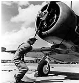
Photo #: 80-G-43935 Aviation Machinist's Mate 3rd Class Violet Falkum turns over the Pratt & Whitney R-1340 radial engine of a SNJ-4 training plane, at Naval Air Station, Jacksonville, Florida, 30 November 1943. This photograph was used in a World War II recruiting poster. Official U.S. Navy Photograph, now in the collections of the National Archives.
